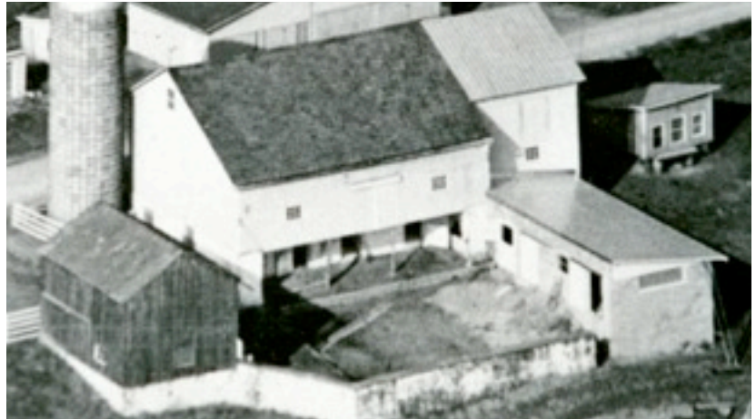
Pre 1953 photograph showing the Pennsylvania forebay bank barn (1844) with posted forebay and asymmetrical roof line.
